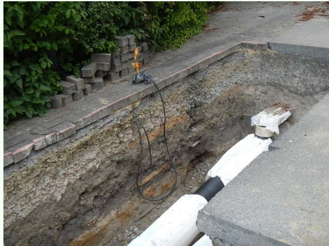
Reconstruction of underground water supply lines in Bielefeld (Germany) (photo: Makowsky)
